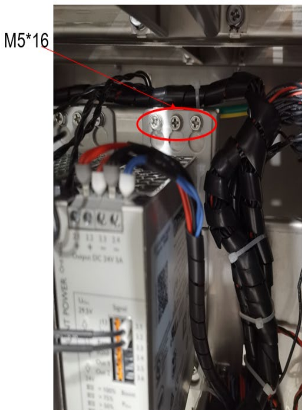
Connection point of small power supply (SP3)
